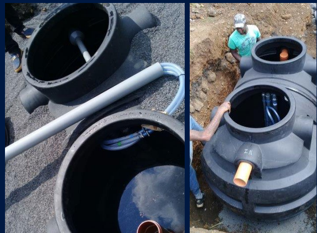
3000 L Small scale Waste water treatment plant
