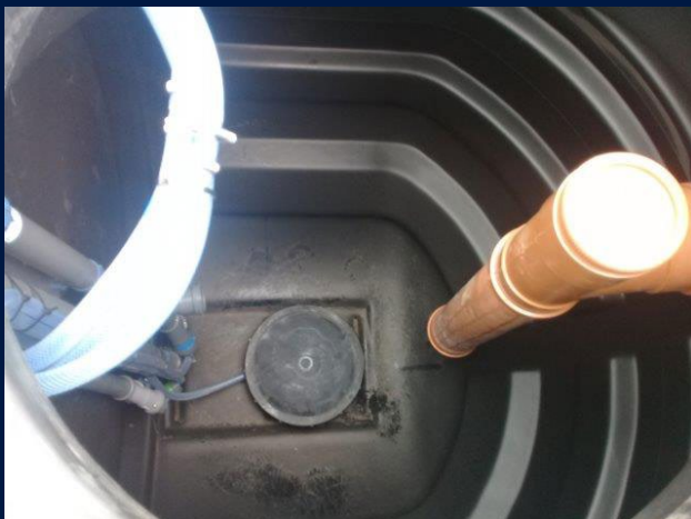
Air Lift Pumping- no submersible pumps
